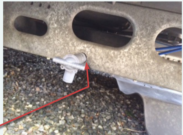
Hole has been drilled to allow for the plumbing fitting
