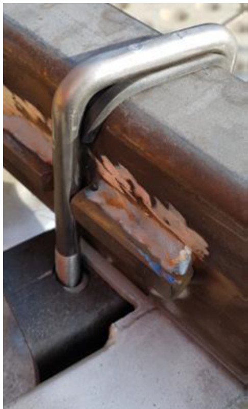
Figure 3-1-7. New front mount of the repaired Trailpro 8x4 and 8x5 trailers
