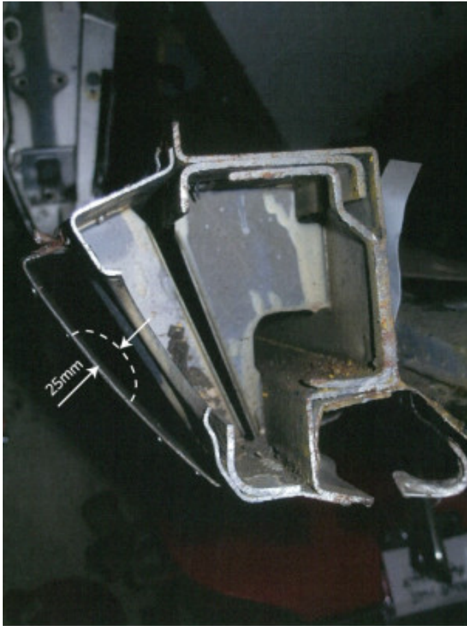
Figure 3-4-1. Outer sills cross section and rocker panels
